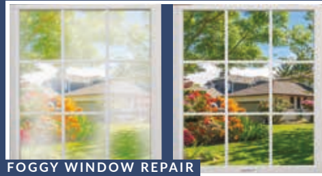
FOGGY WINDOW REPAIR
