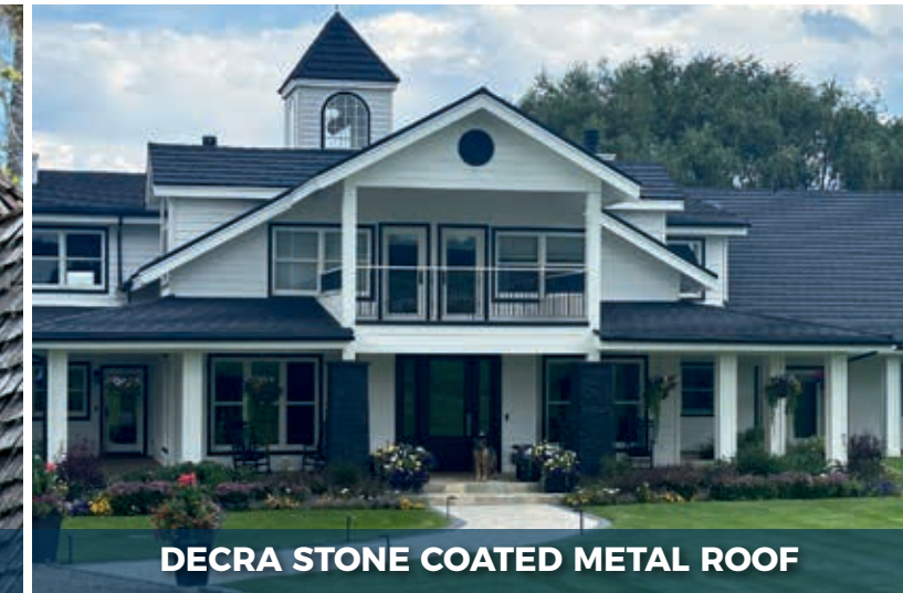
WEATHER DAMAGED WOOD SHAKE ROOF
